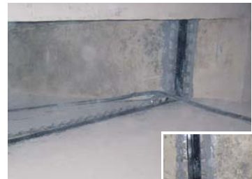
Sealing of a construction joint in a container for potable water, corner shaped, with AMEX ® -10 MONO Seal
