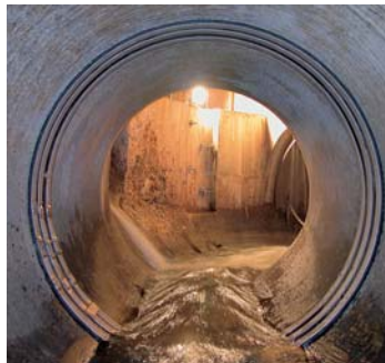
Sealing of a potable water pipe with AMEX ® -10 MONO Seal, 366 mm wide with inflating water
