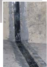
Sealing of a construction joint in a container for potable water, corner shaped, with AMEX ® -10 MONO Seal
