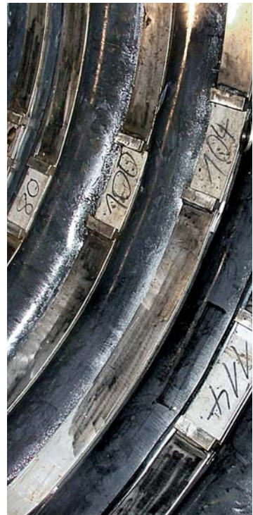
Detail showing a AMEX ® -10 VARIO installation under strong water pressure from outside
